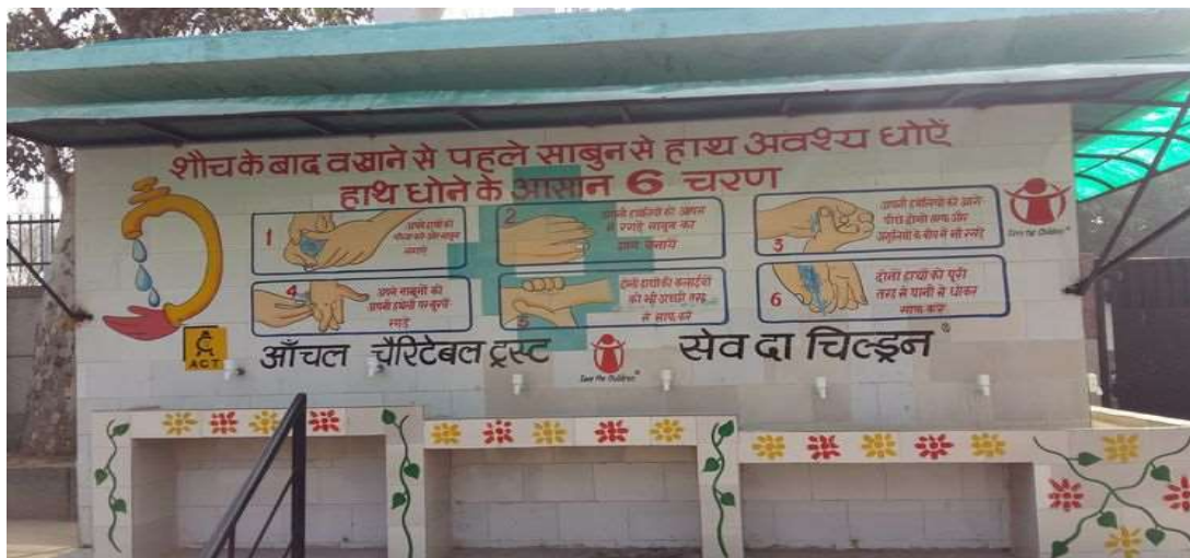
Rehabilitated Drinking Water Point at Government School
